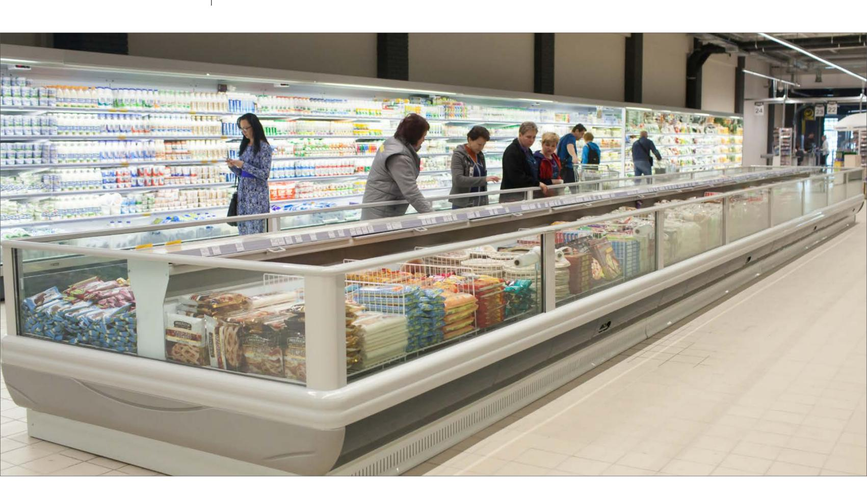
Low-temperature Nautilus cabinets with energy saving covers and inner LED lighting of volume
